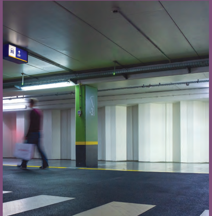
Underground car park with permanent steel sheet pile walls at Hopmarkt shopping center, Aalst, Belgium
