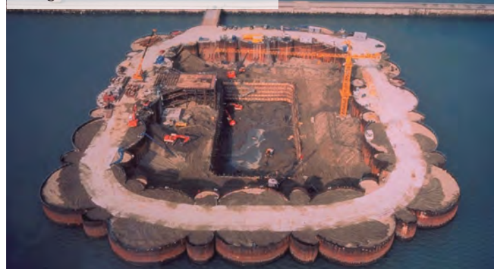
Bridge construction, South Korea
