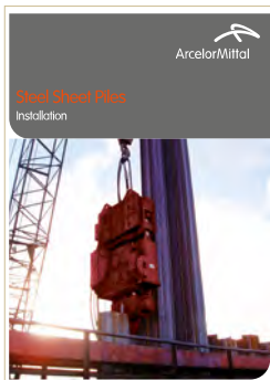
Installation of sheet piles GB, DE, FR
