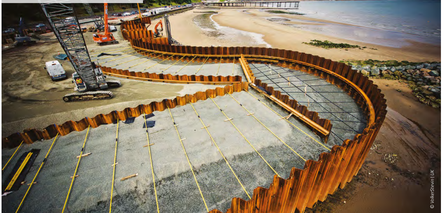
Coastal defense project, Colwyn Bay, UK
