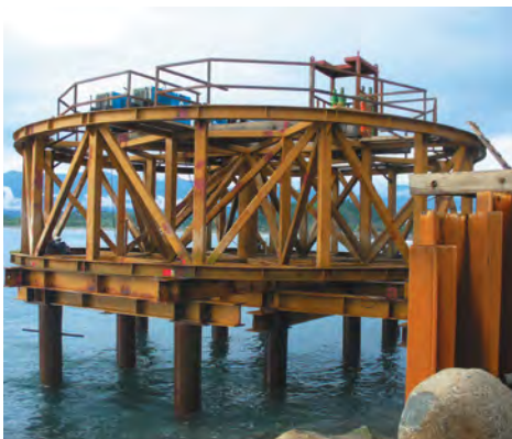
1. Installation of template
