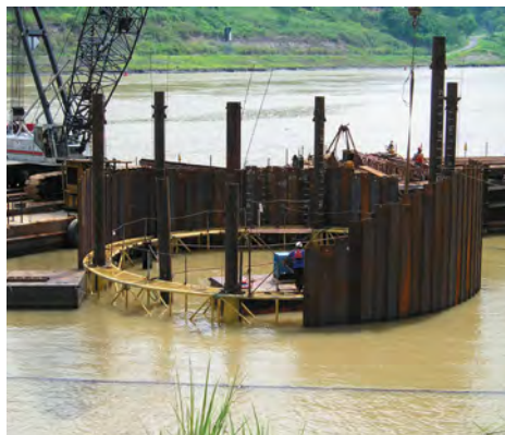
2. Threading until cell closure
